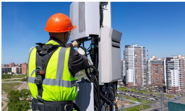
Figure 9: A small cell can be placed on a building in downtown areas, shopping centers, and college campuses.
